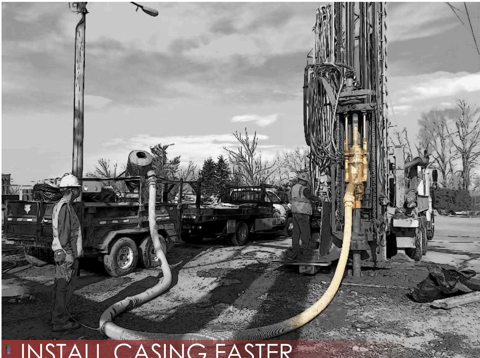
CD140 putting in water well casing
