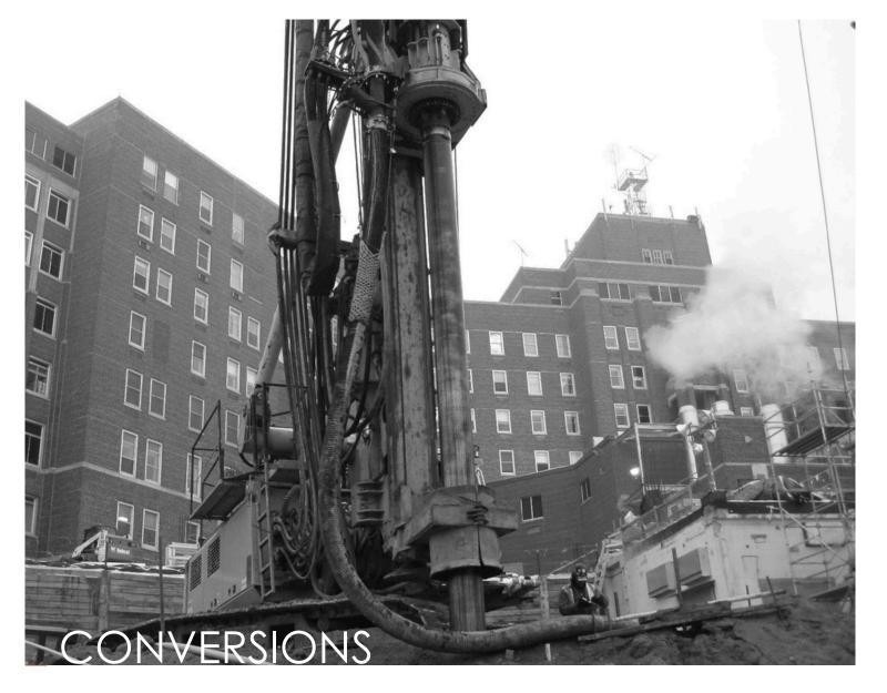
Because older rigs are not capable of using reverse circulation systems effectively, we have found it necessary to modify them for RC. By applying our experience and custom components, we are able to fabricate the proper tooling to work most efficiently with the rig.
