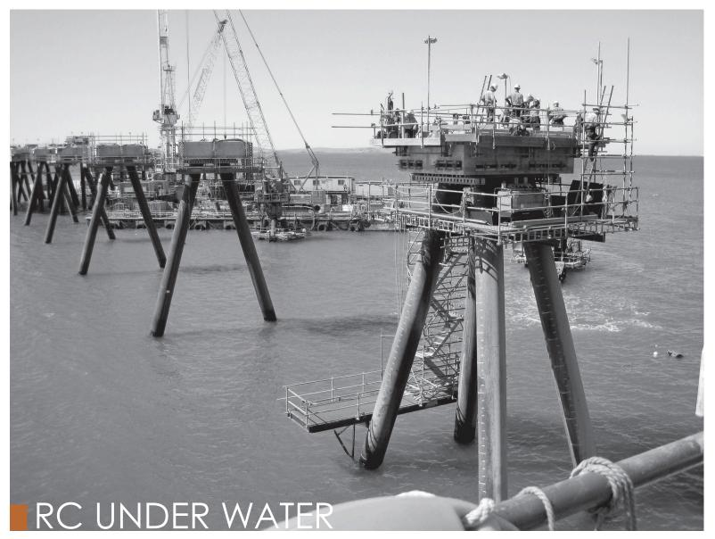
When drilling in water, additional back pressure from high water depths can cause serious degradation in DHH performance. Routing water up the center in RC significantly minimizes the 'Flood-out-Factor' by reducing the back pressure.
